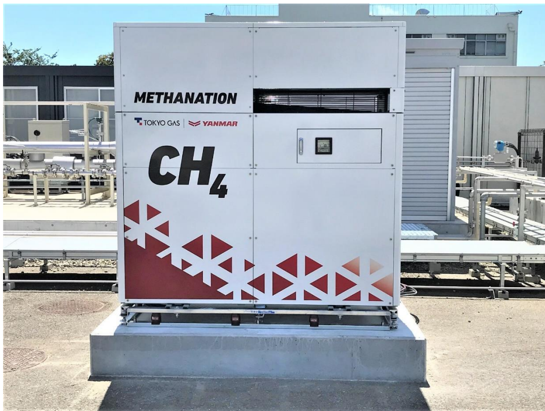
Methanation gas compatible micro cogeneration demonstration unit.
