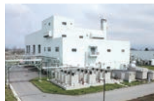
Biogas micro cogeneration system CP Series (for biogas made from sewage)
